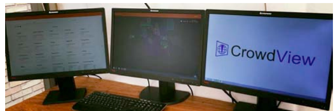
figure 2: CrowdView setup in control room.
